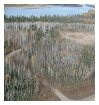
figure 8. A well-design pit with a doglegged access and vegetated buffer zones.
