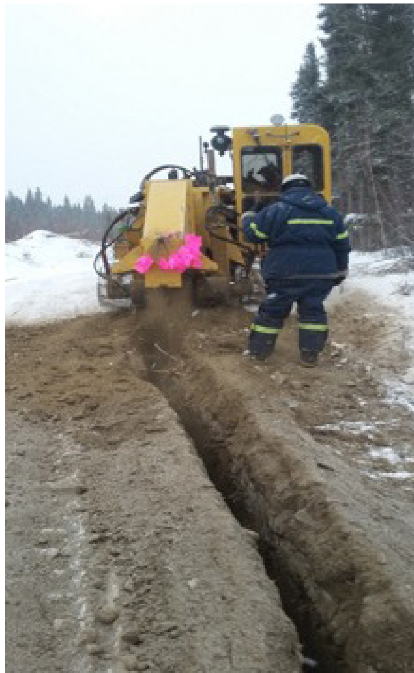
Figure 7: Trenching and laying the Fibre optic cable along the Mackenzie Valley, March 2016. Review Board photo.
