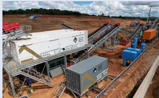
Example: Construction of Modular Process Plant
