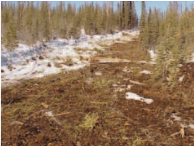
FIGURE 41. Brush can be rolled back across steep slopes to prevent erosion.
