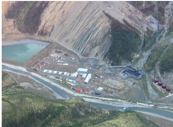
Canadian Zinc Corporation's Prairie Creek mine site.
